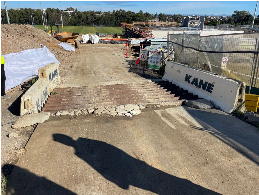
Rumble grid and hardstand at main Site access.
