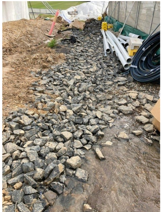
Swale drain following immediate rectification works on 21 May 2024 showing debris removed.
