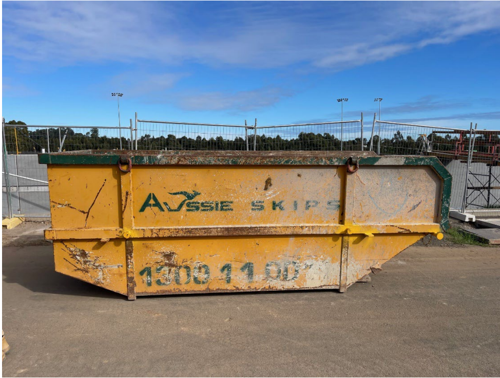
Waste bins available and well within capacity.
