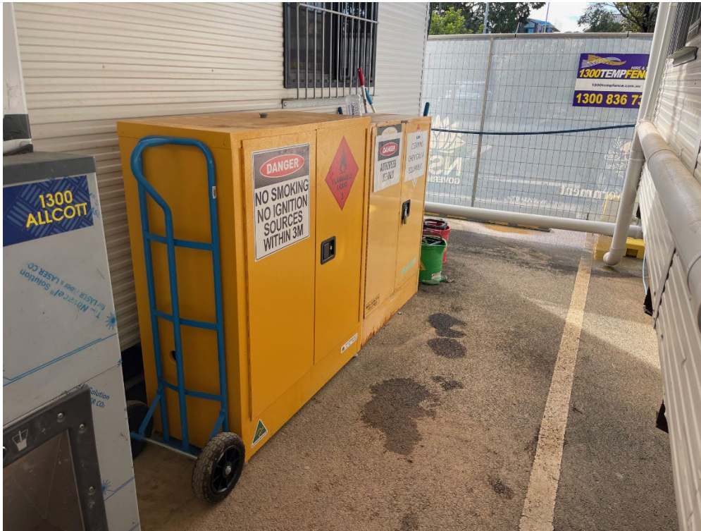
Dangerous goods cupboard with appropriate signage.
