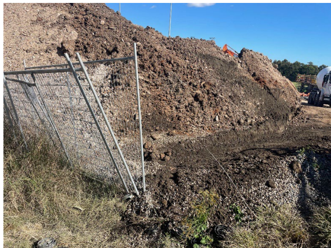
Tree protection area following immediate rectification works on 21 May 2024. Showing dewatering of tree area and a temporary drainage pathway formed via relating the stockpile.
