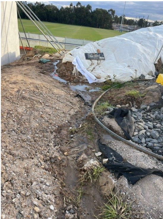
Swale drain following immediate rectification works on 21 May 2024 showing debris removed.
