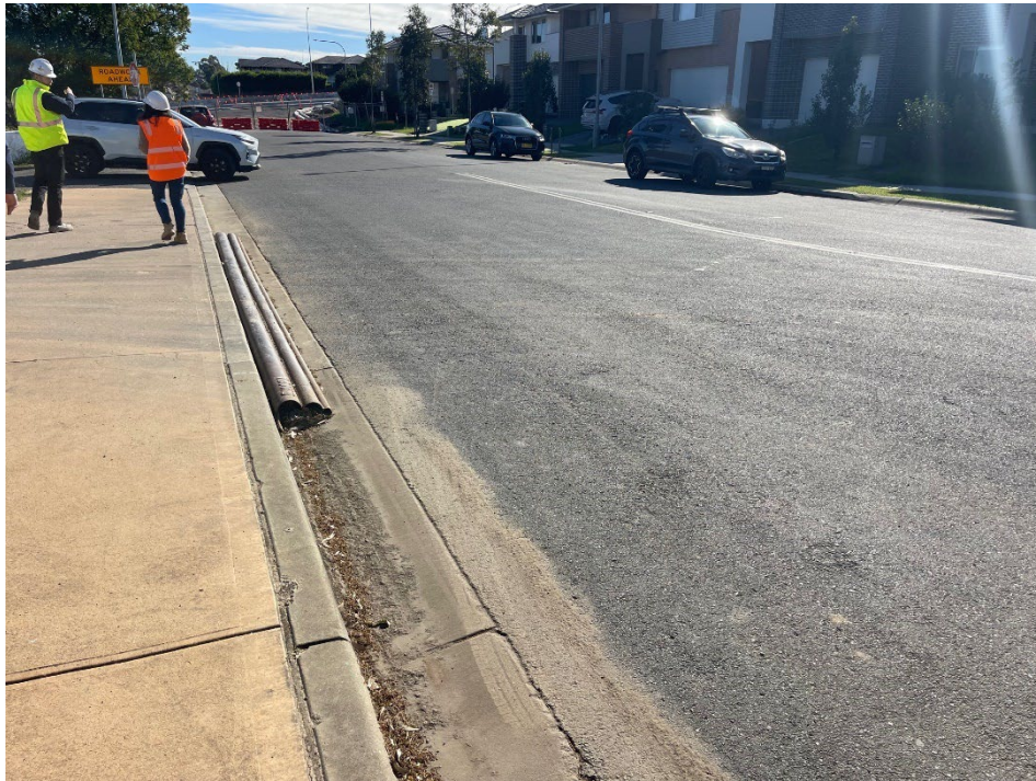
Main Site vehicle access. No sign of mud tracking on public roads.
