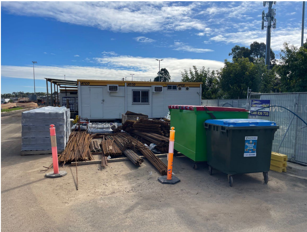
Laydown area kept generally clean and tidy.
