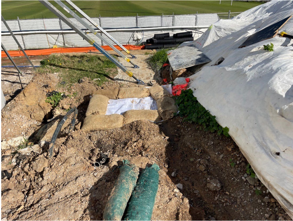
Protection of pit drain.
