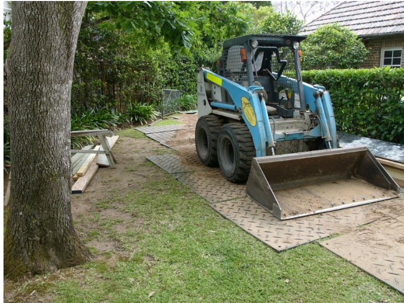
Figure 4 – Showing typical detail for truck mats.
