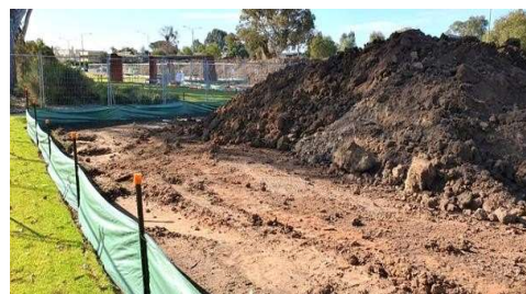
Figure 1. Silt curtain used to control sediment loss
