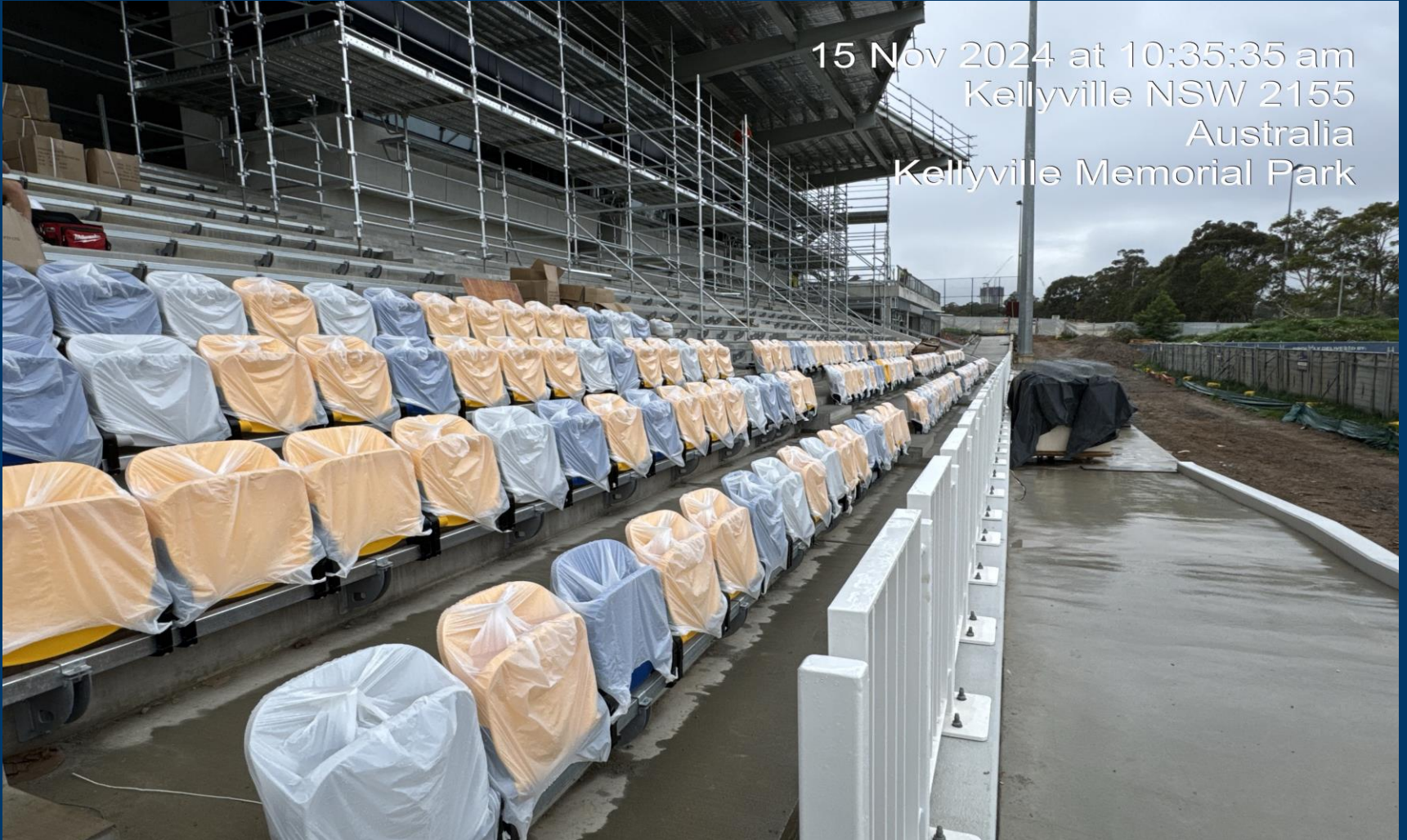
Building A – Grandstand Seating Installation (South)
