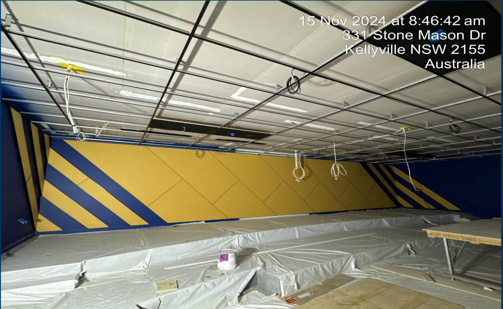
Building B – Acoustic Panels Installation (LGF Theatre Room)
