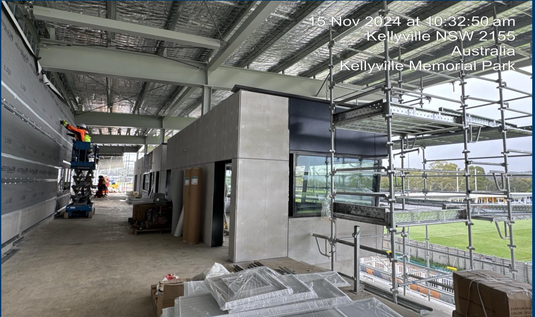
Building A – Window Installation (Coaches & Media Boxes)
