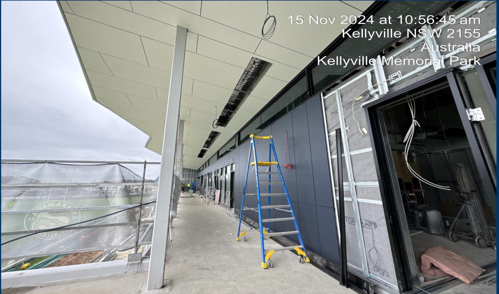
Building B – Painting to Western Elevation
