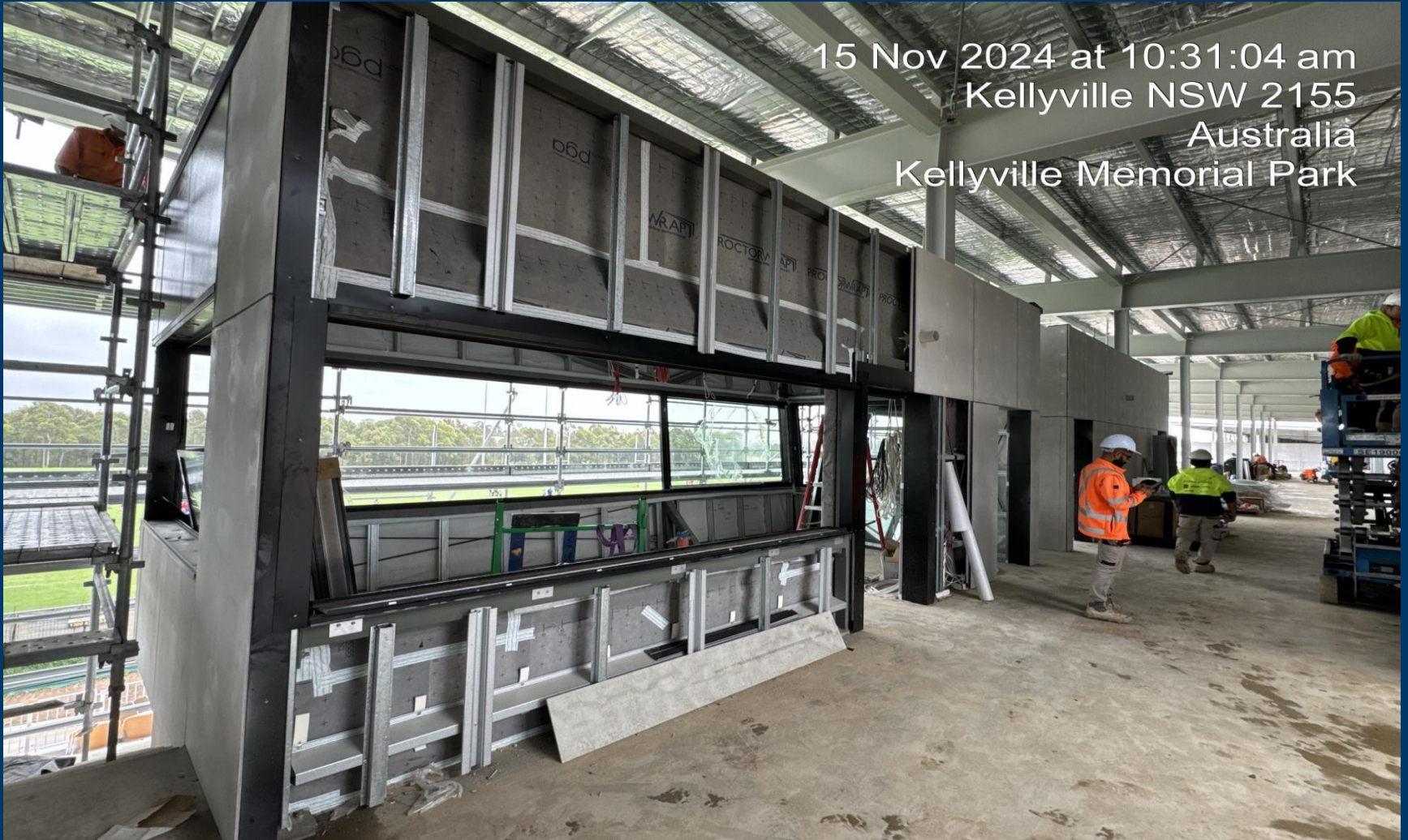
Building A – External Sheeting (Coaches & Media Boxes)
