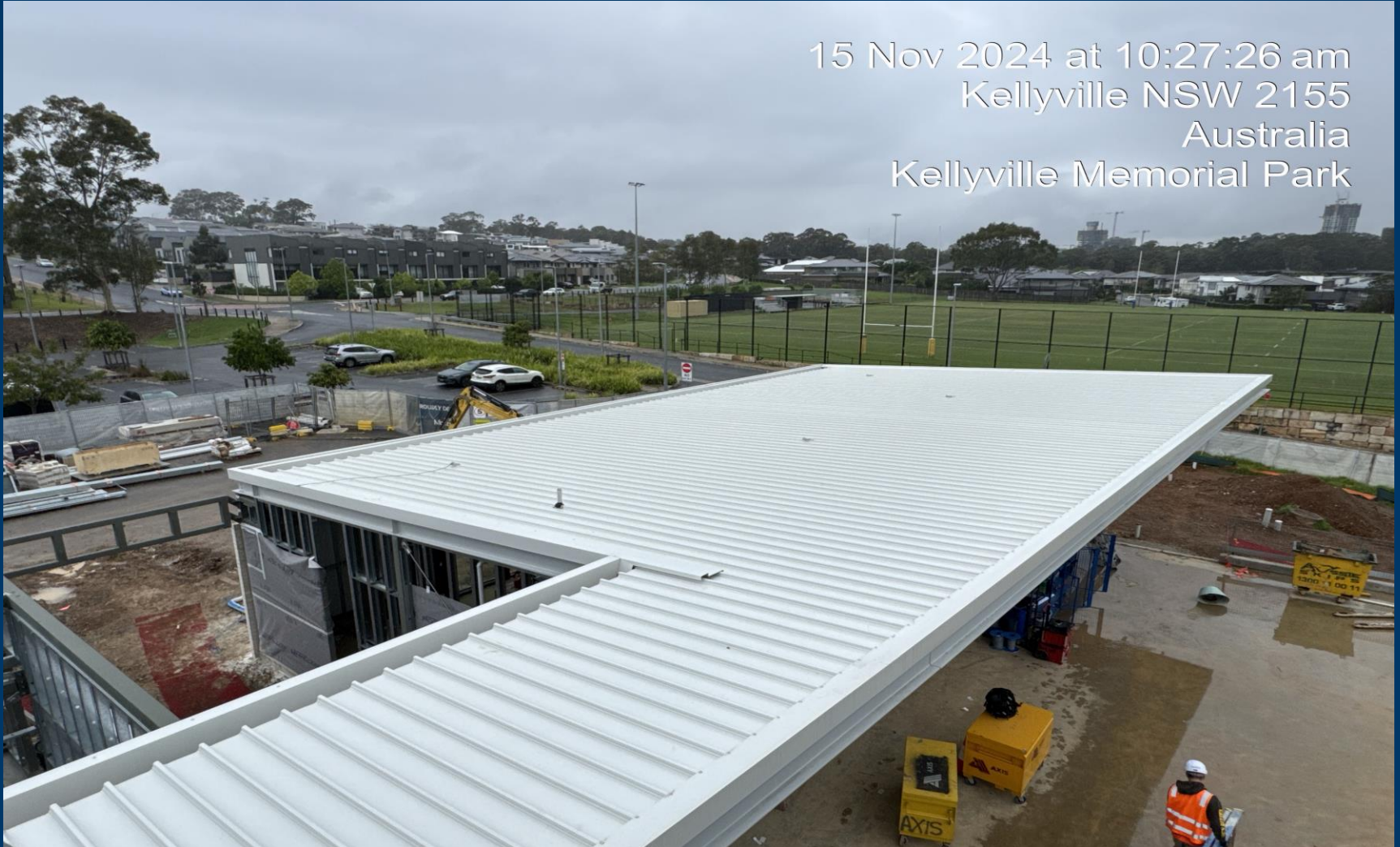
Building A – Roofing Complete (Tenancy Area)
