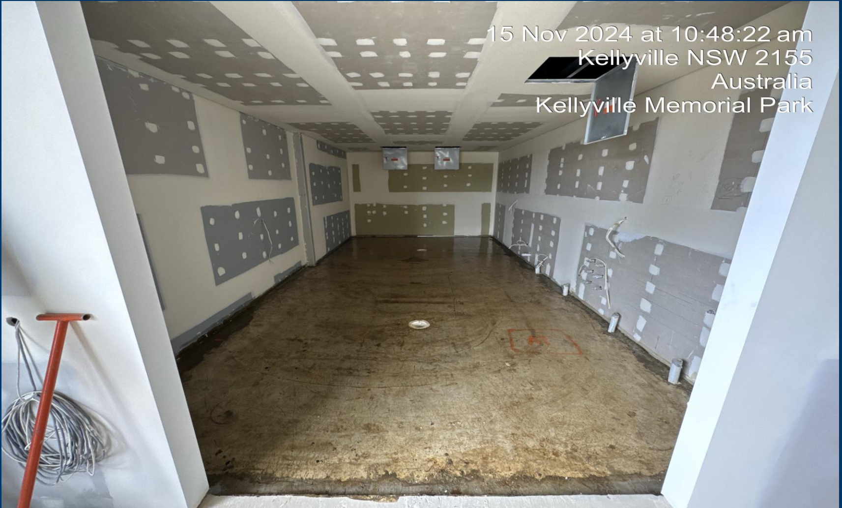
Building B – Floor Preparation (GF Pour 1)
