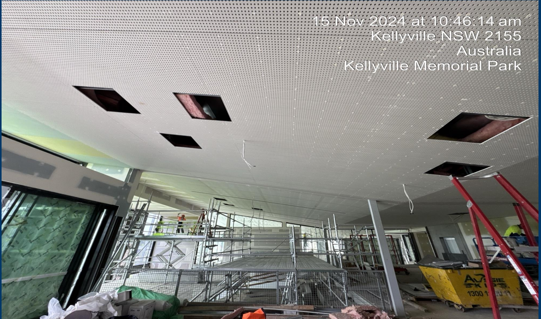
Building B – Setting and Sanding Ceiling (GF Pour 2)
