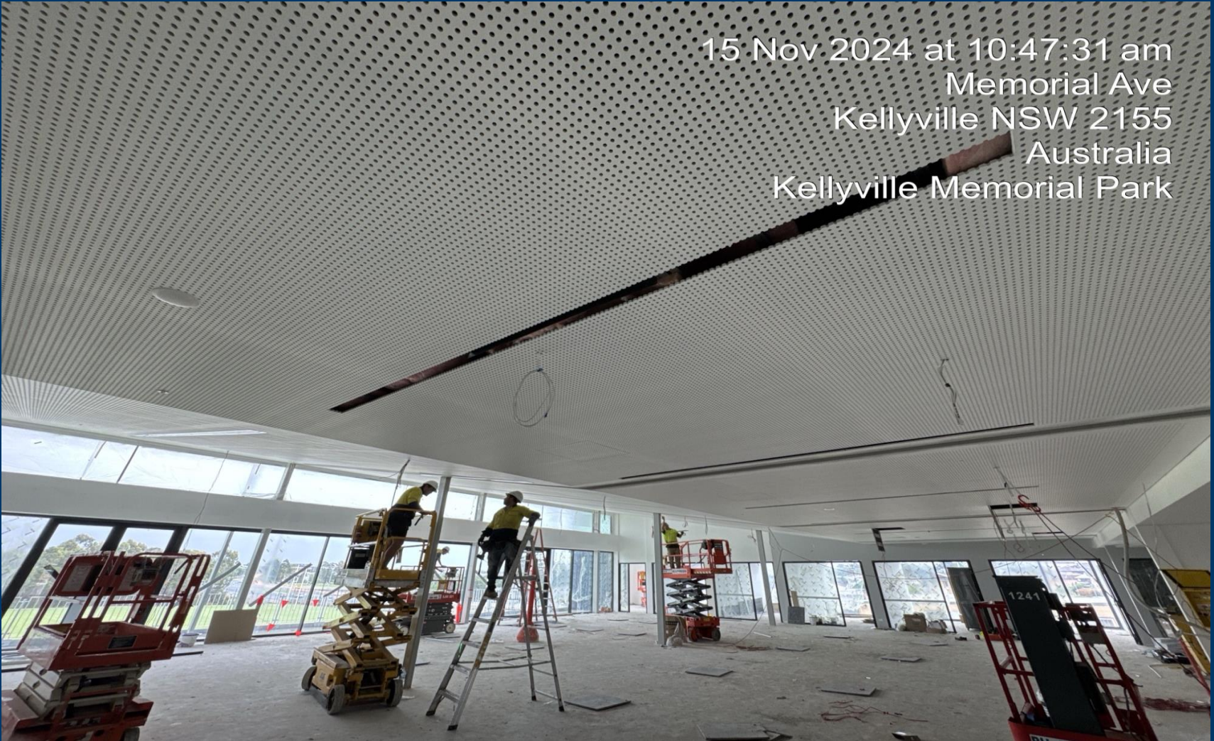
Building B – 1 st Coat of Paint (GF Ceiling Pour 1)
