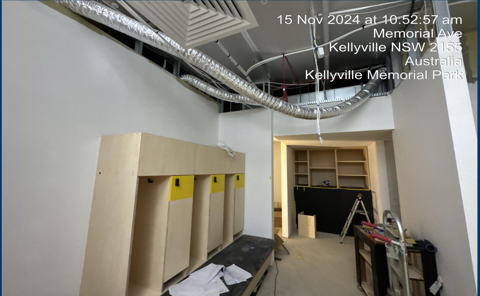
Building B – Joinery Installation (LGF Pour 2)
