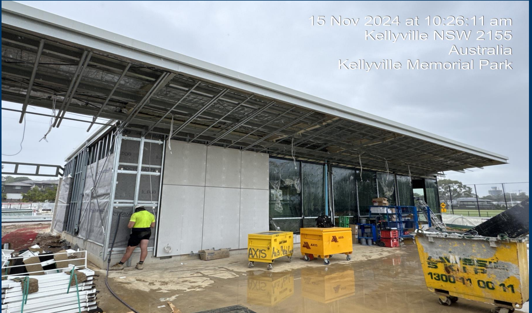
Building A – Sheeting External Walls (Tenancy Area)
