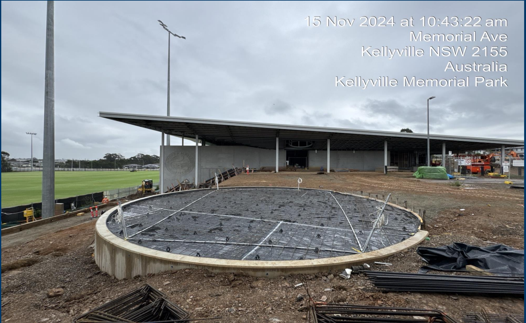
Steel Fixing to Meeting Place Circle
