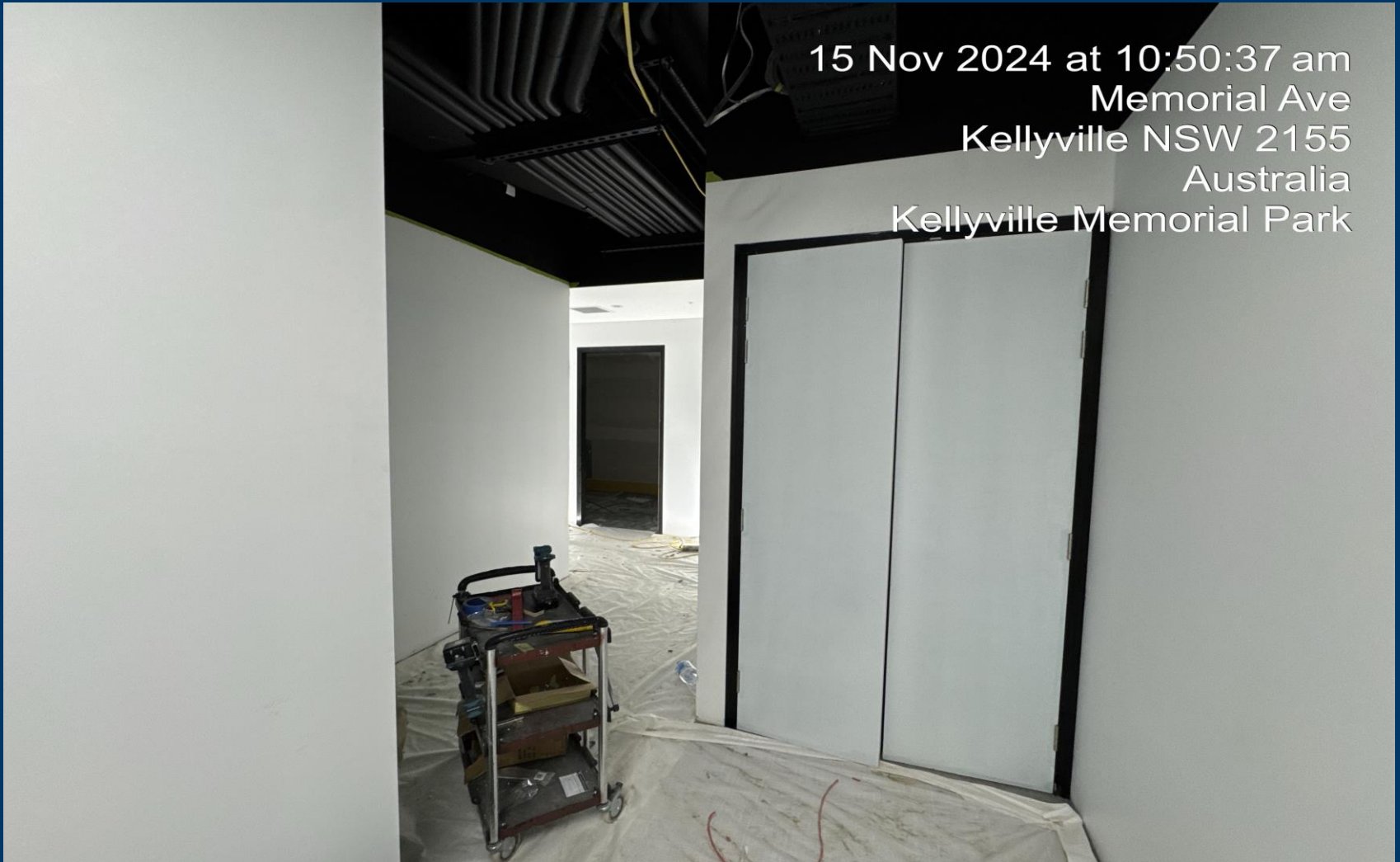
Building B – Door Hardware Installation (LGF Pour 1 Area)
