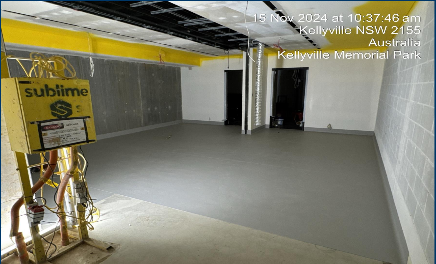
Building A – Vinyl Installation (LGF Area)
