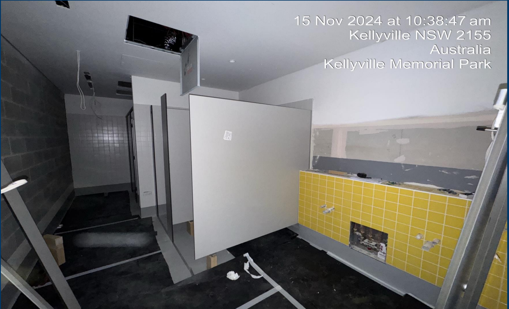
Building A – Installation of Toilet Partitions (LGF Area)
