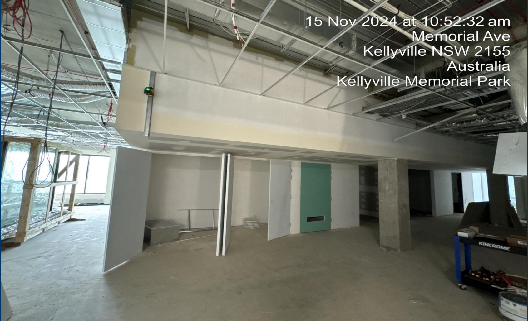
Building B – Door Hardware Installation (LGF Pour 2 Area)
