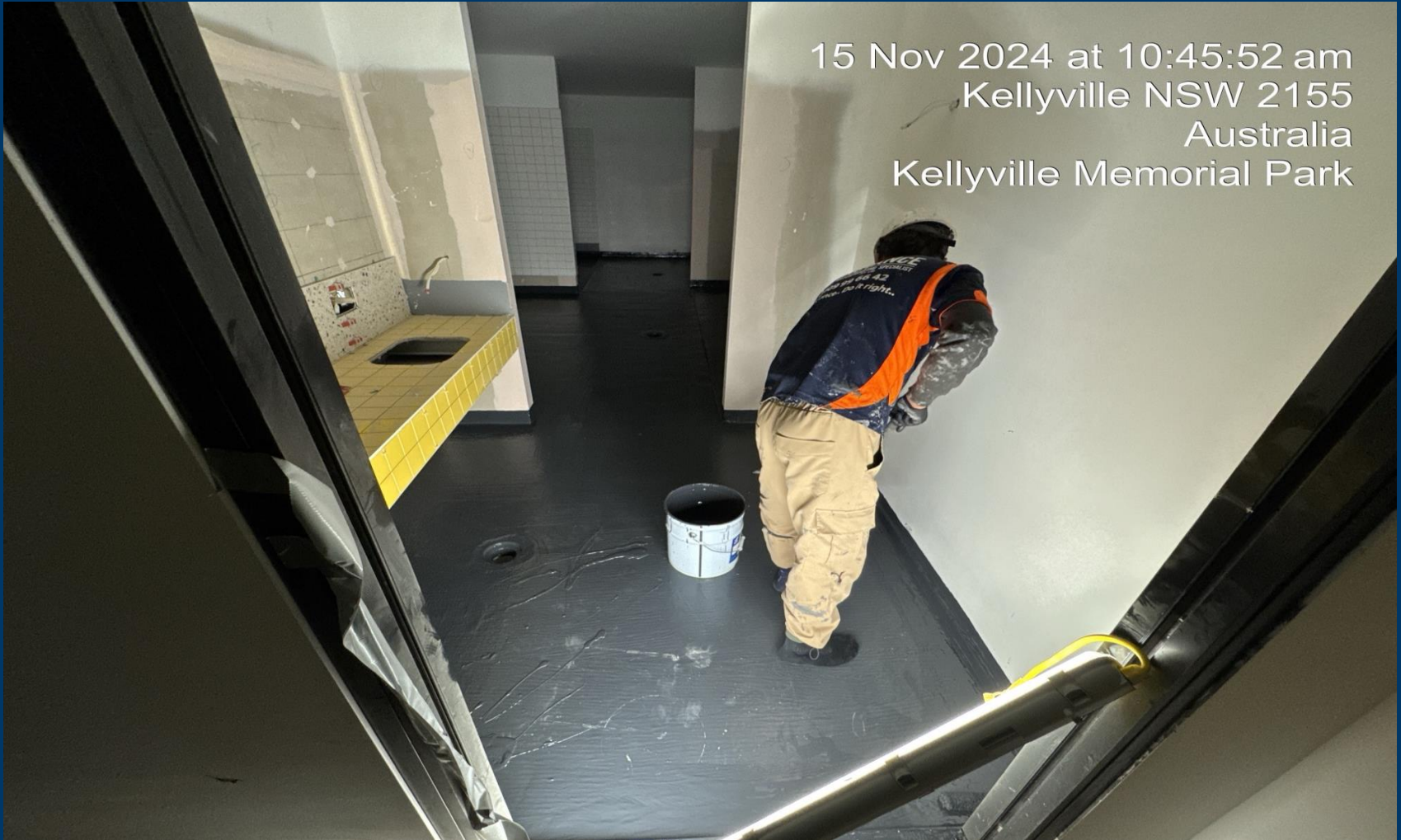
Building B – Waterproofing (GF Wet Areas)
