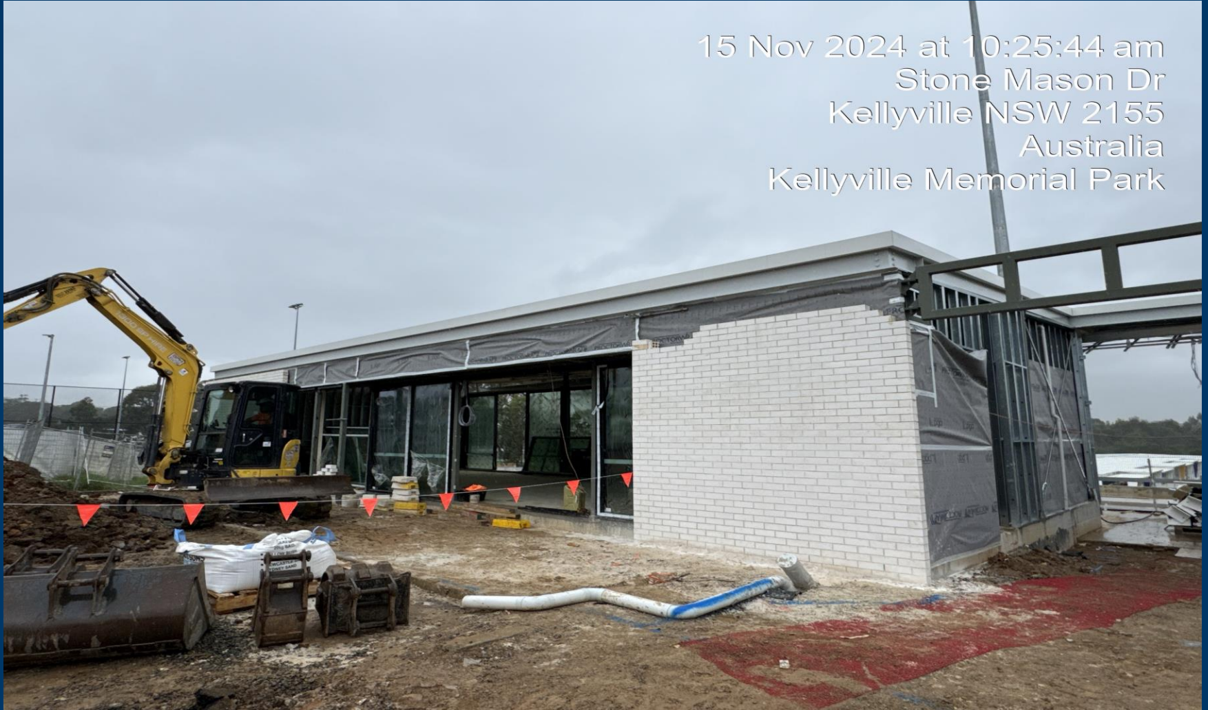
Building A – Brickwork (Tenancy Area)
