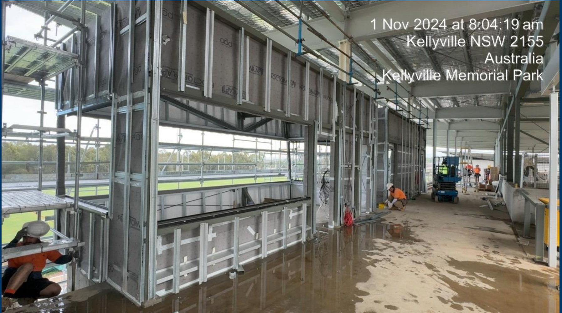
Building A – Internal and External Sheeting (Media & Coaches Boxes)
