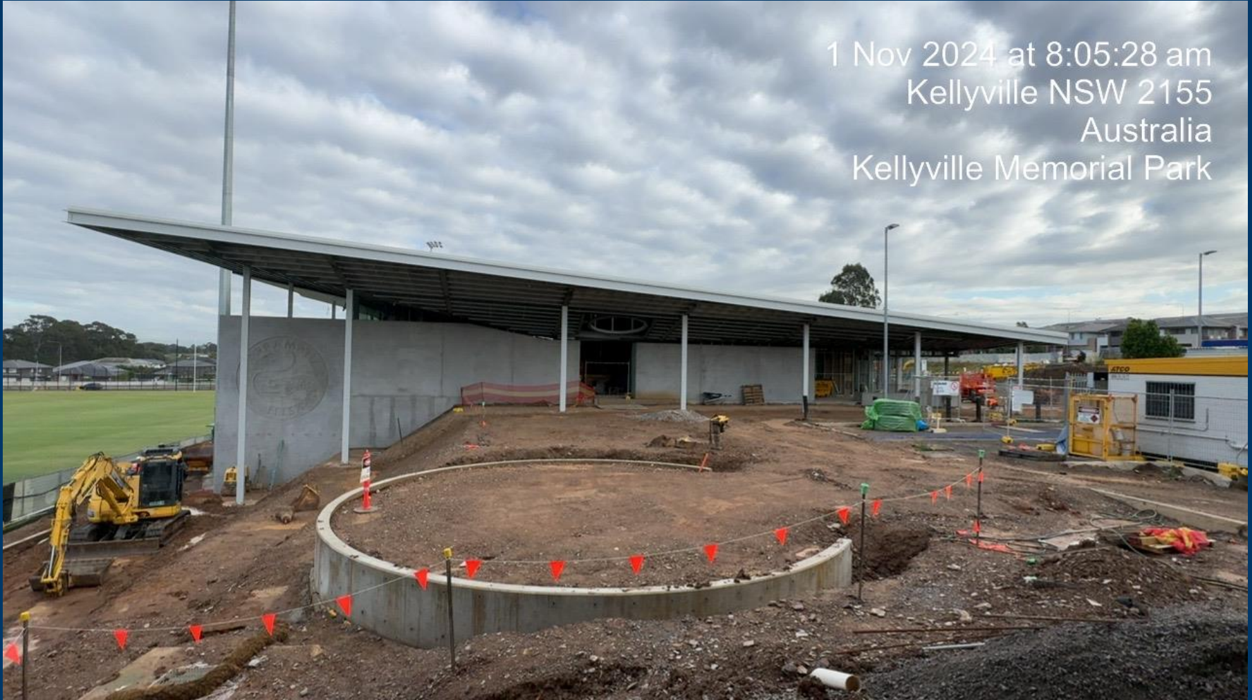
Backfilling of Meeting Place Area
