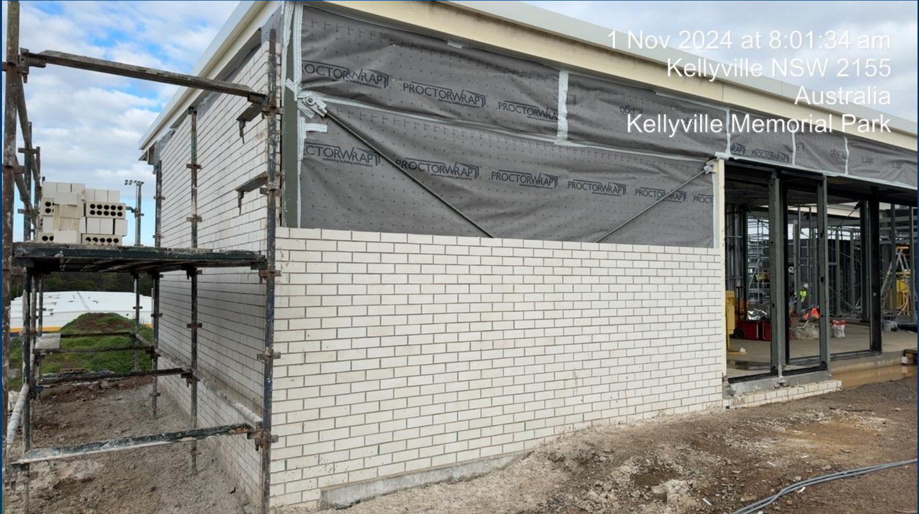
Building A – Brickwork (Tenancy Area)
