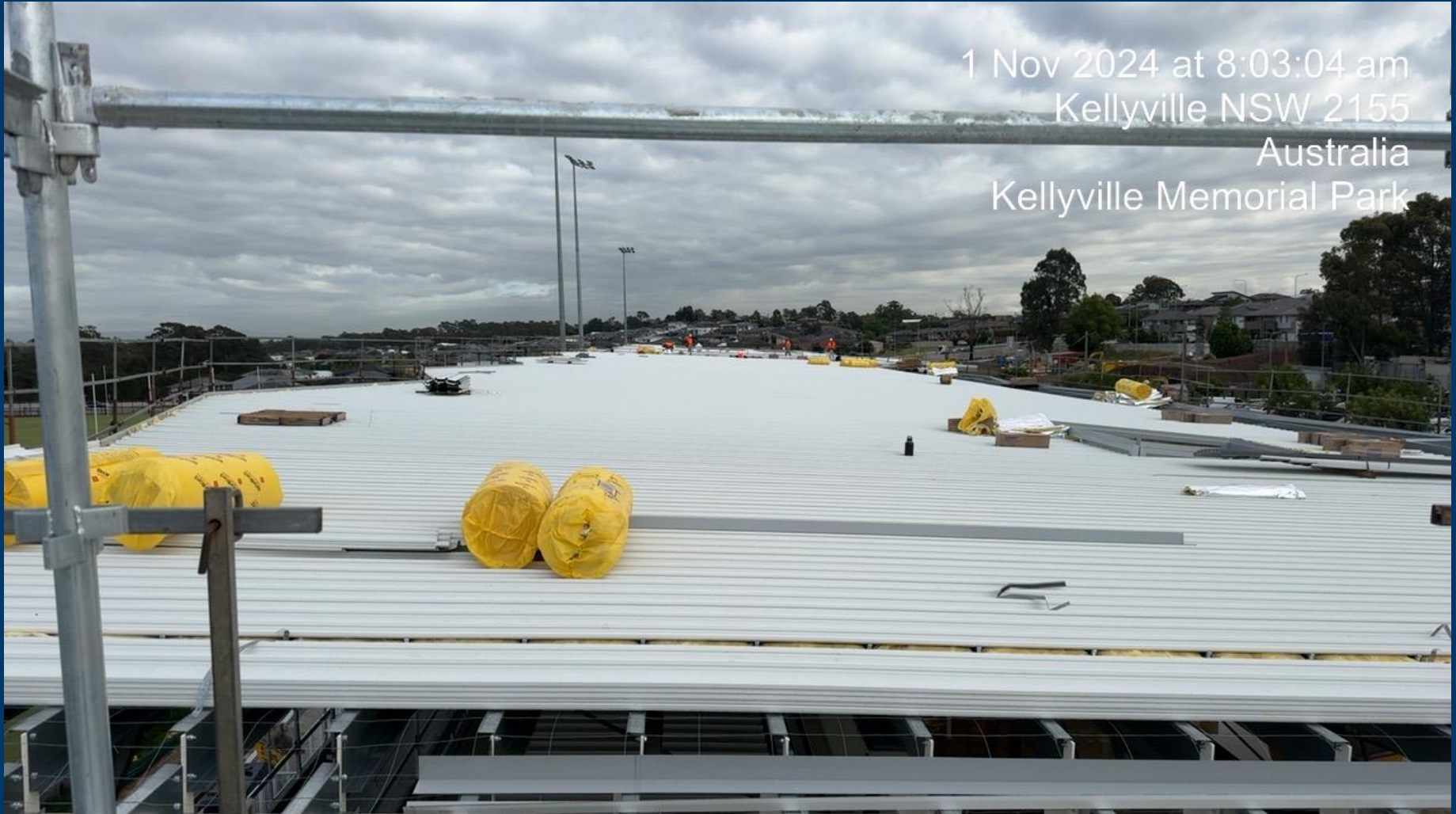
Building A – Roof Sheet Installation
