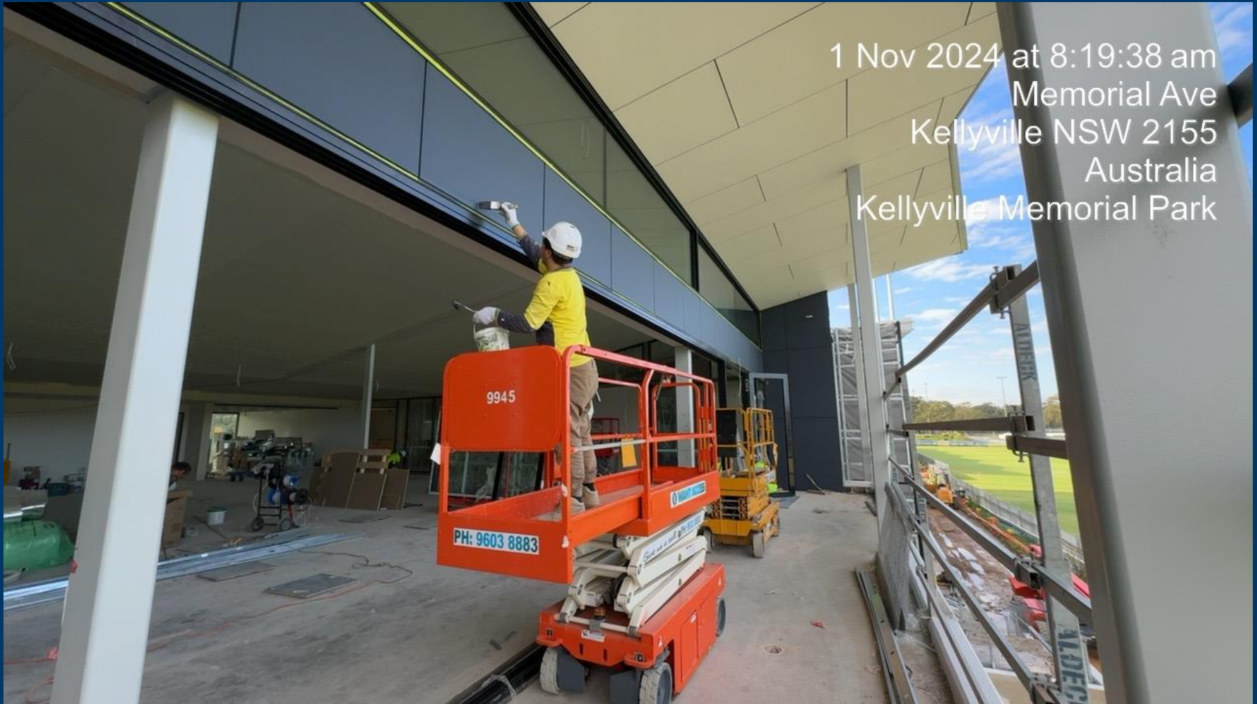
Building B – Western Elevation (GF Pour 1 Painting)
