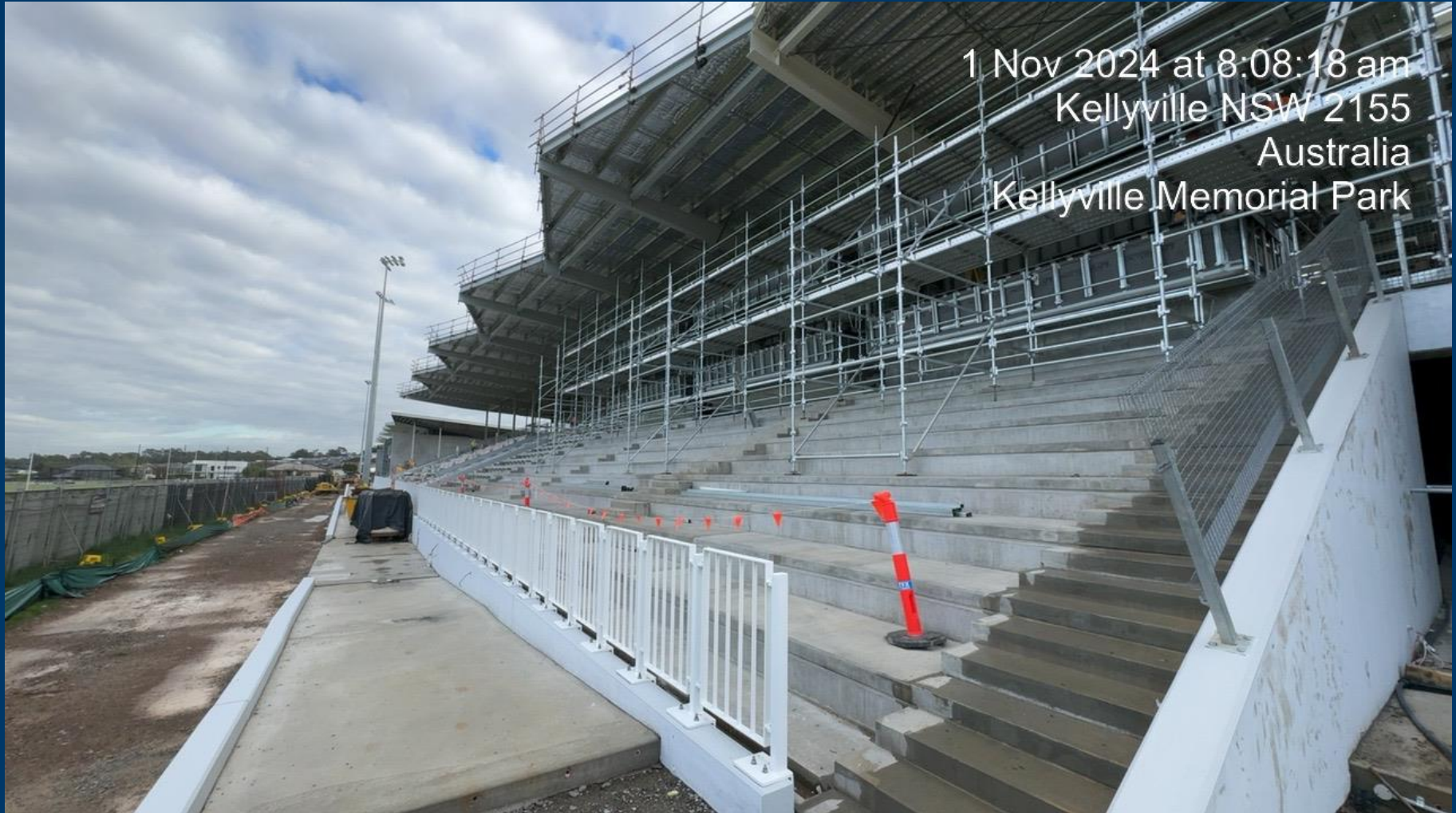
Building A – Handrail Installation (Seating Plats)
