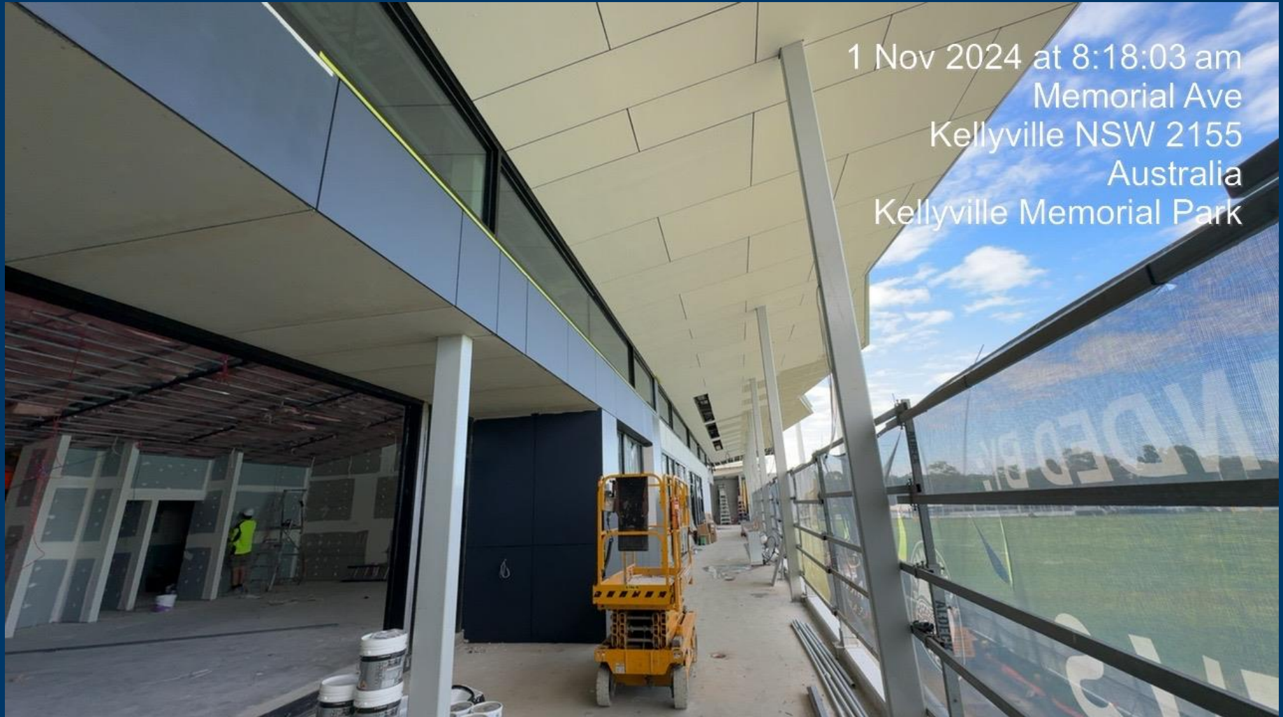
Building B – Western Elevation (GF Pour 2 Painting)
