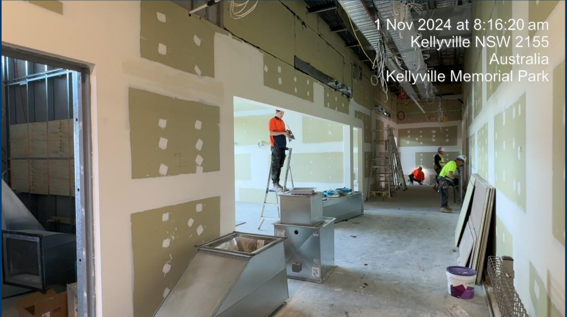
Building B – Sheeting and Setting Walls (GF Pour 3)
