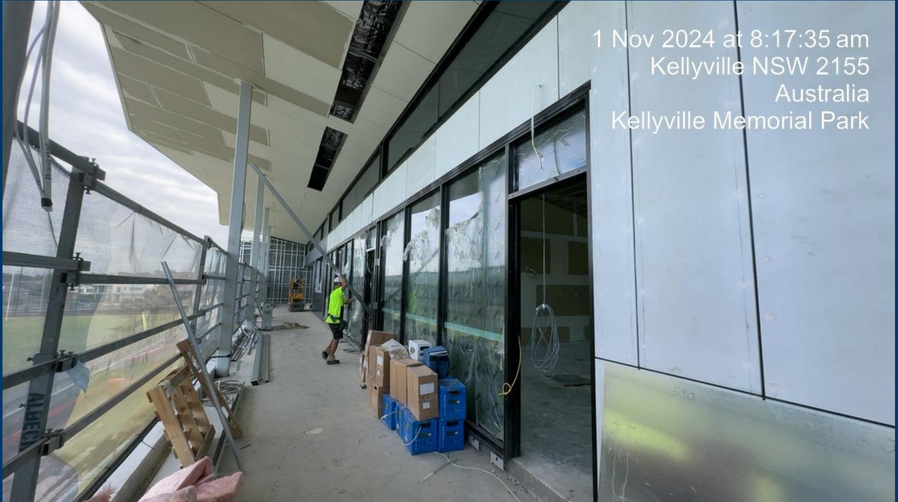
Building B – Low Level & High-Level Window Installation (GF Pour 3)
