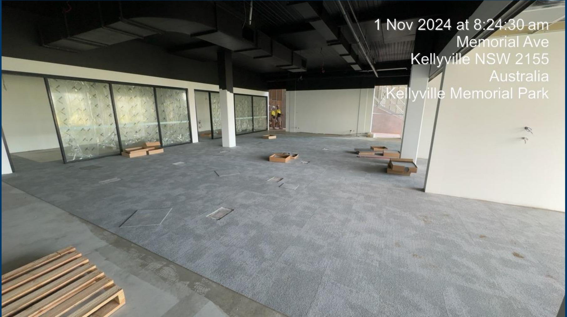
Building B – Installation of Carpet Tiles (LGF Pour 1)
