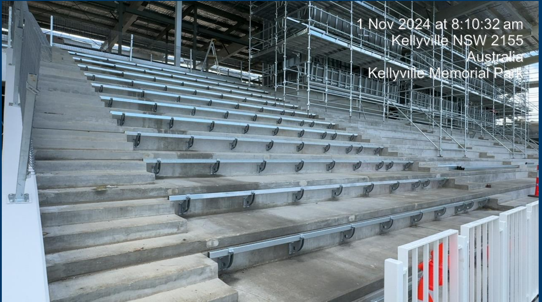
Building A – Installation of Grandstand Seating
