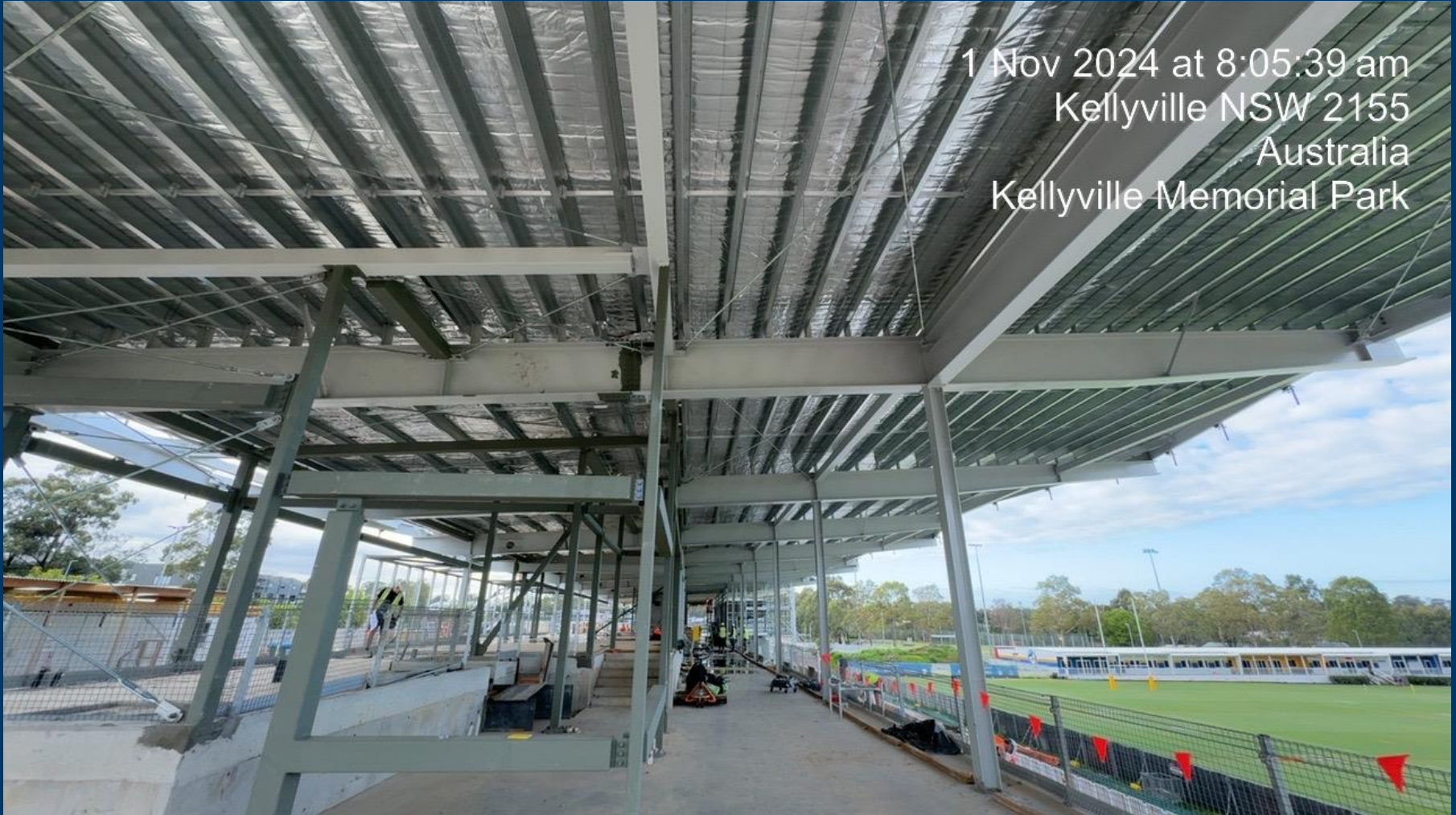
Building A – Completion of Roof Insulation
