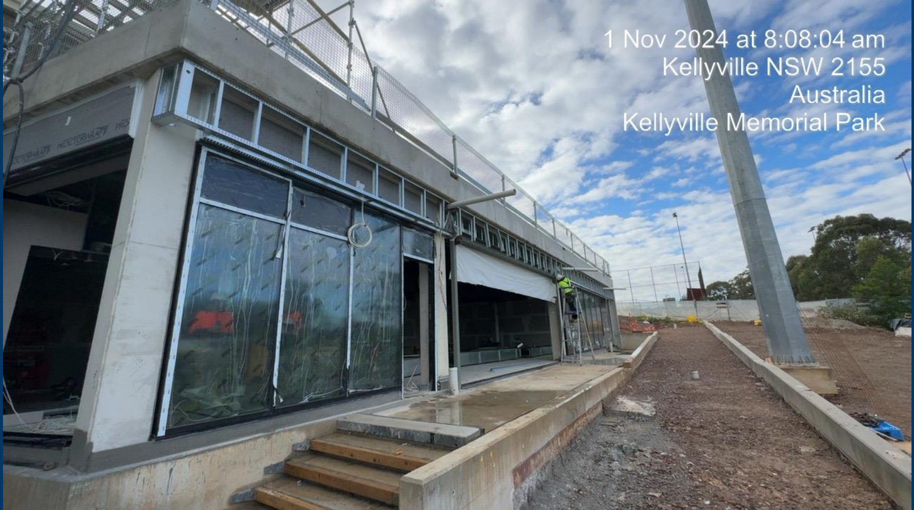
Building A – Installation of Windows (LGF Gym)
