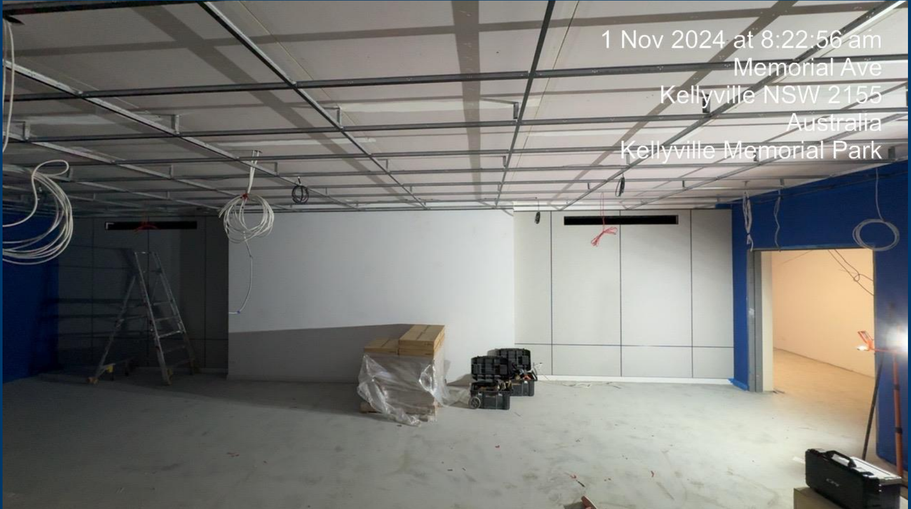
Building B – Installation of Acoustic Wall Panelling (LGF Theatre Room)
