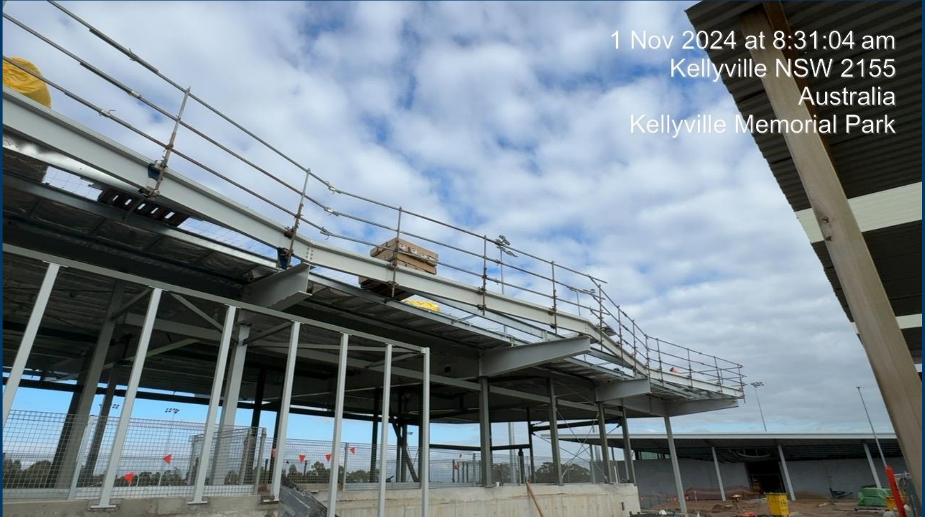
Building A – Roof Handrail Installation
