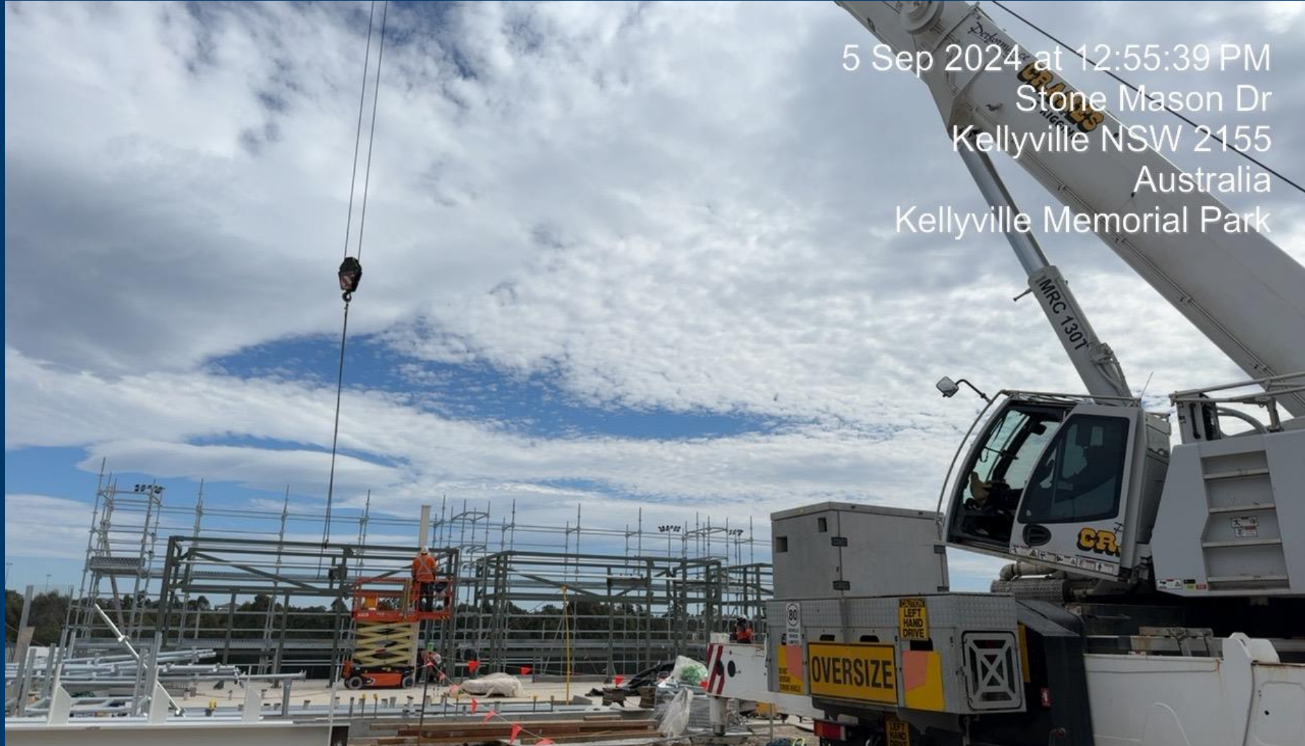
Building A- Structural Steel Installation to Coaches Box
