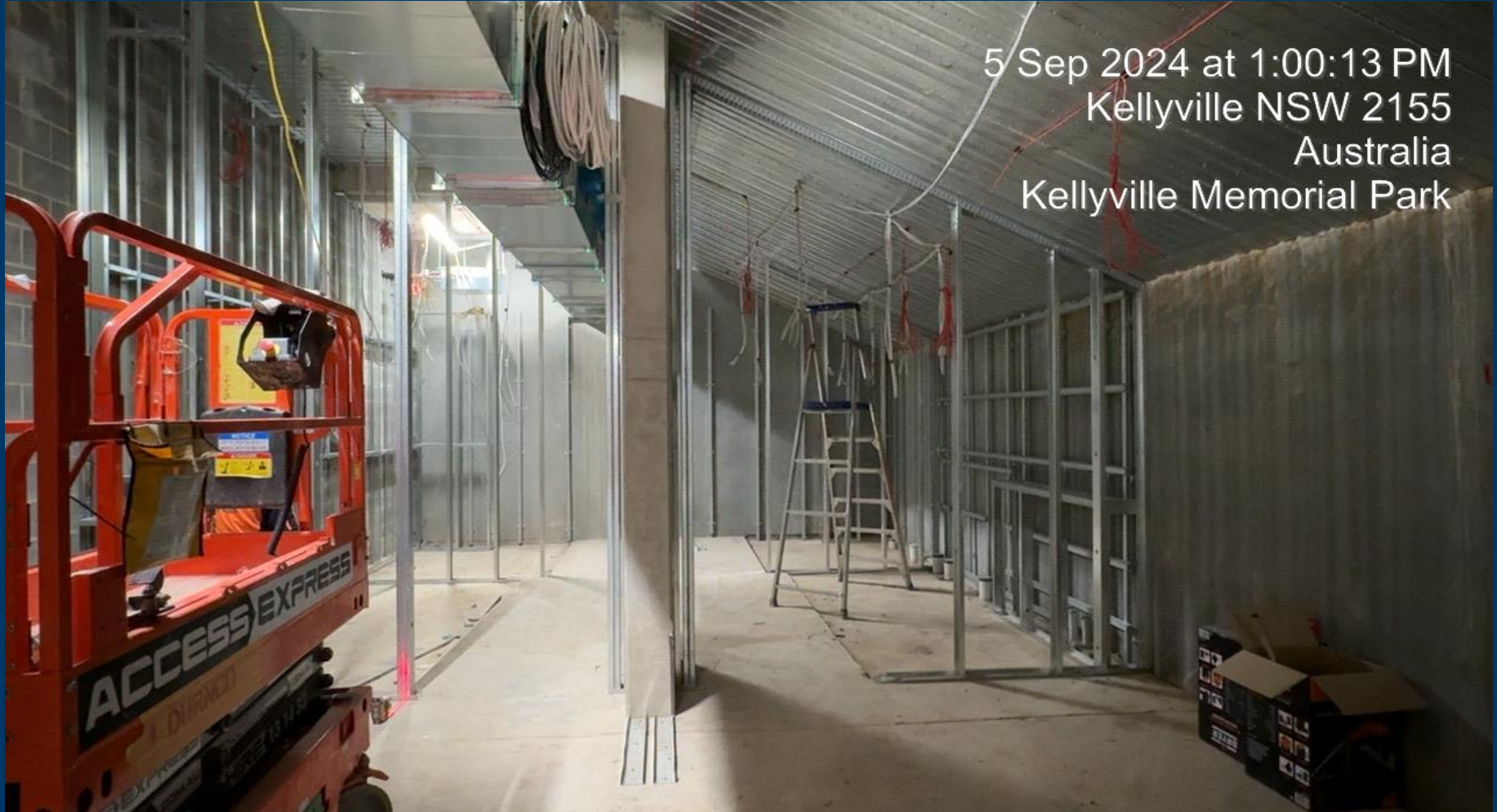
Building A – Framing to Change 2 LGF
