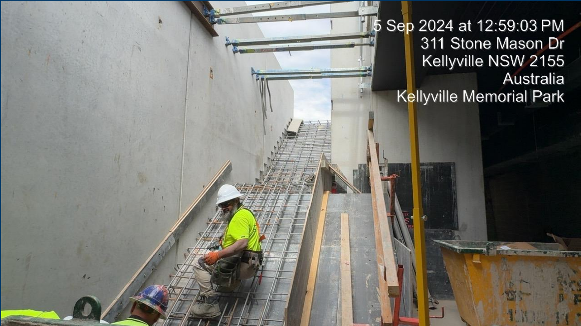
Building A- Formwork and Steel fixing to Stair 1
