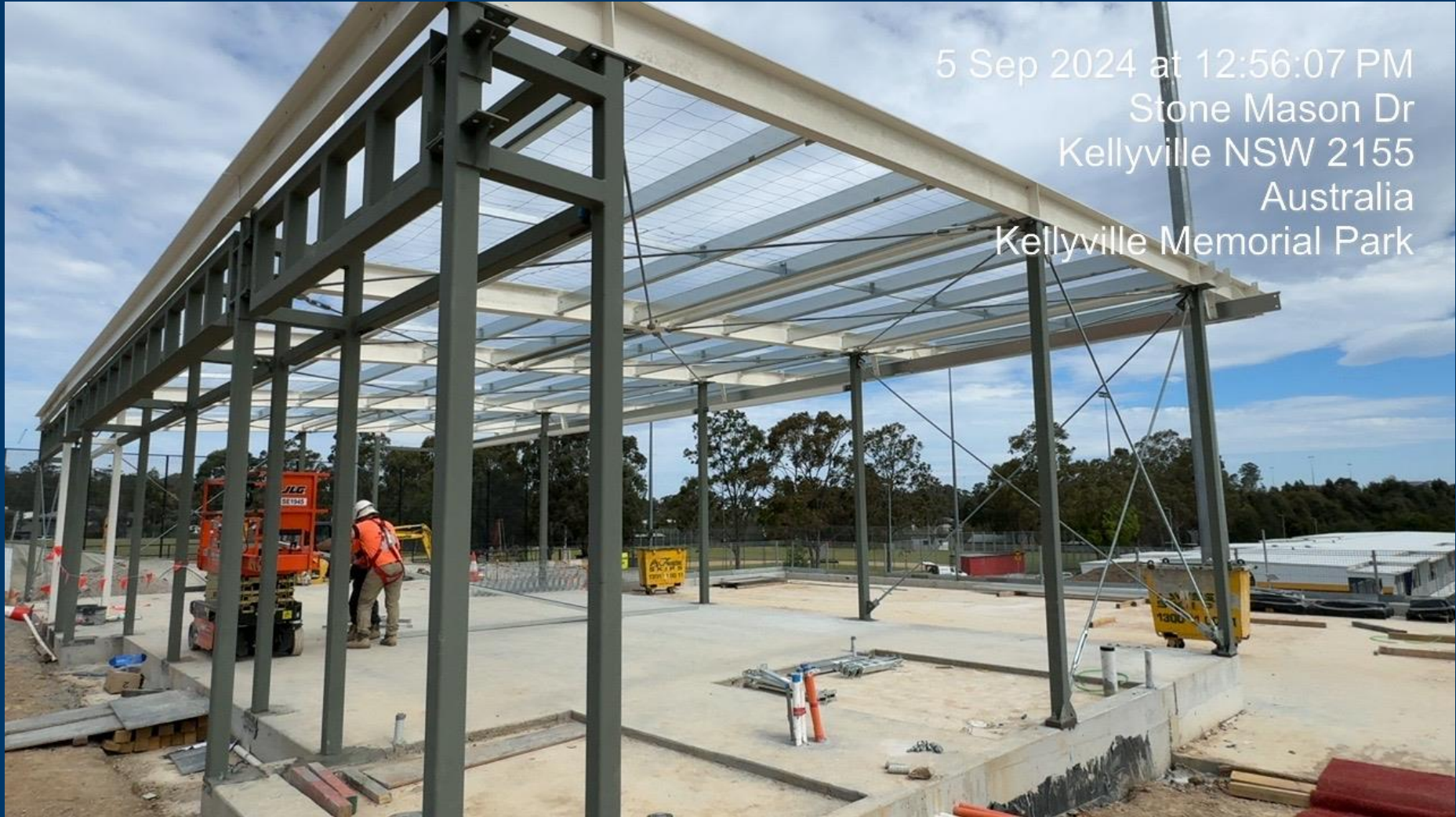
Building A- Roof Mesh to Tenancy Area
