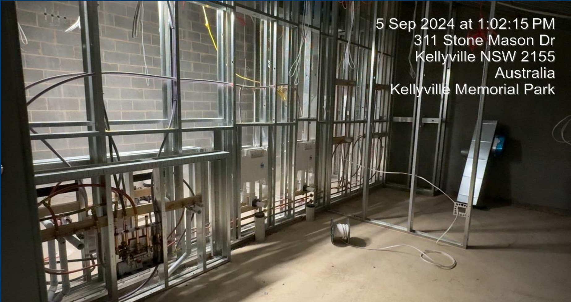
Building A – Services Roughin Male Bathroom LGF
