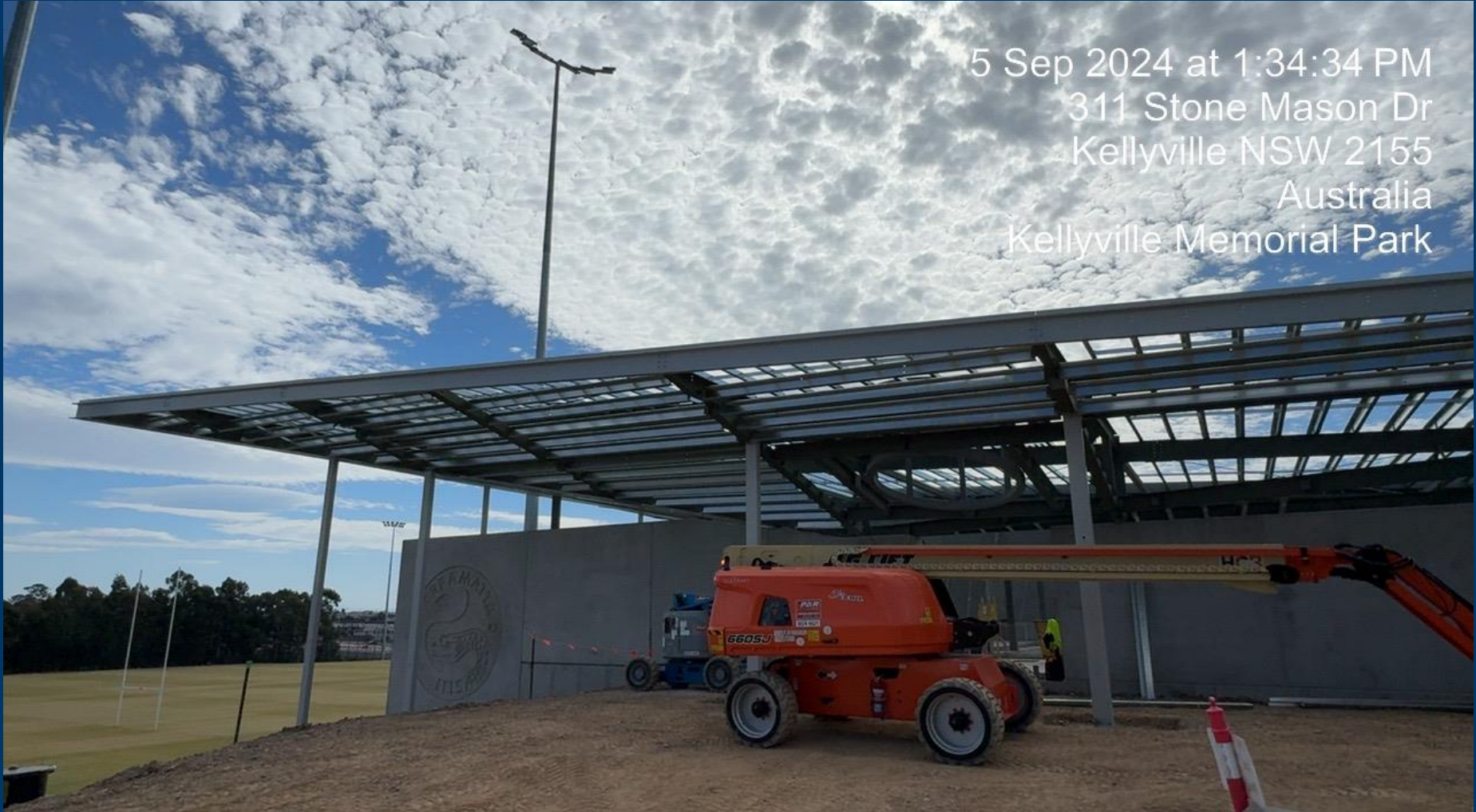
Building B – Completion of Structural Steel
