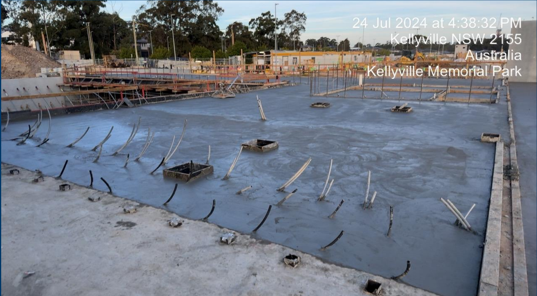
Building B – Upper Floor Suspended Deck Pour 3
