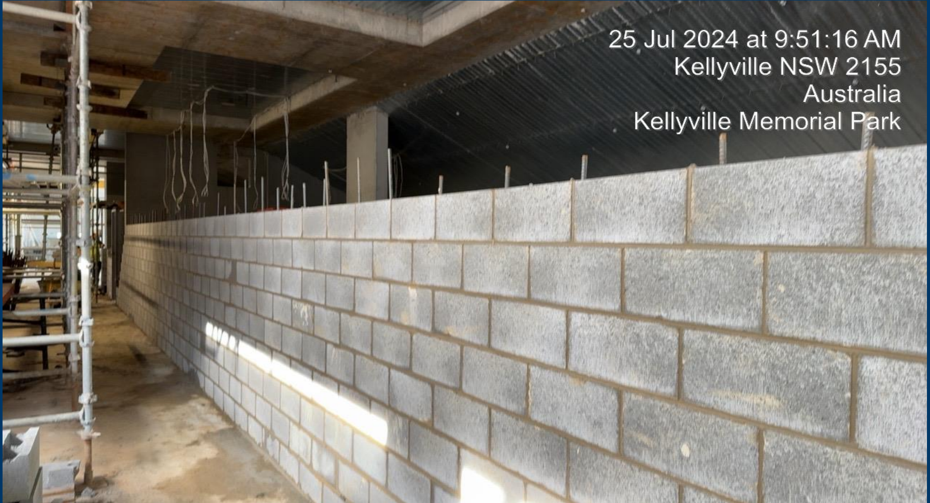
Building A – Blockwork installation Lower Ground Floor
