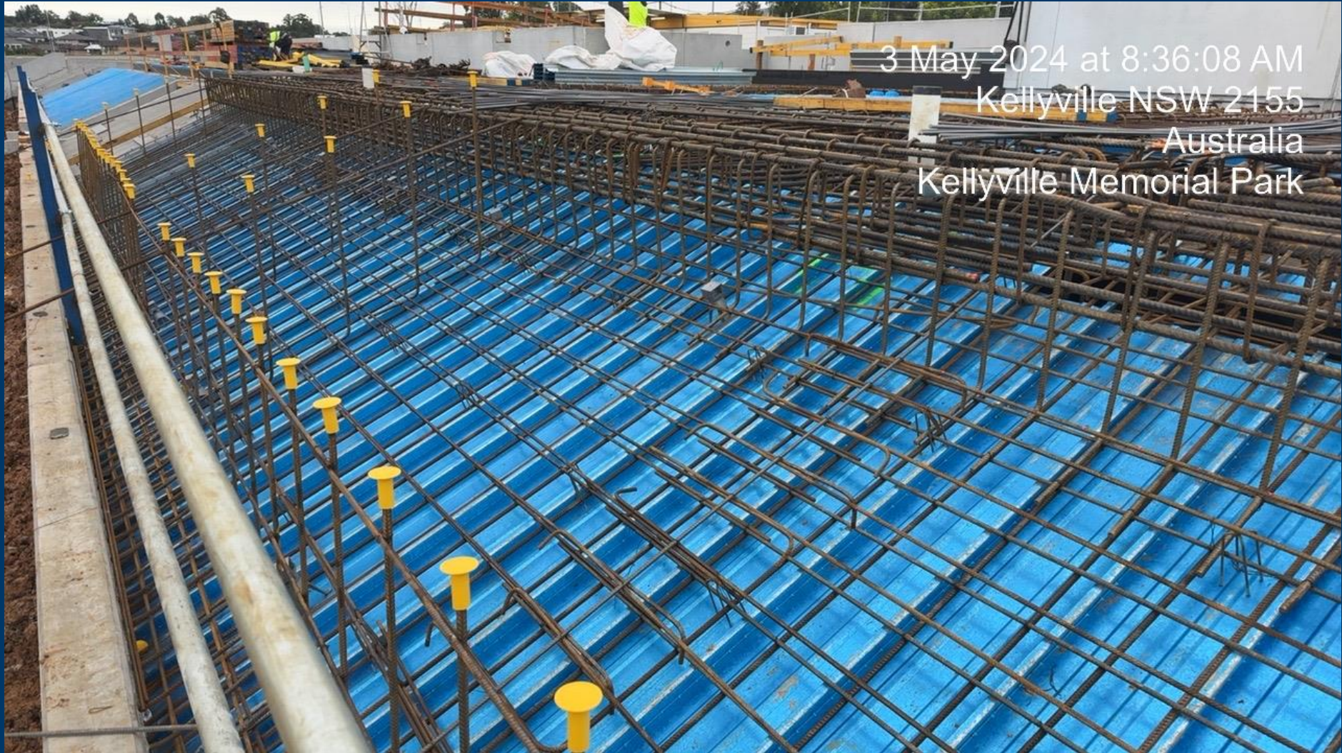
Building A – Rake soffit
