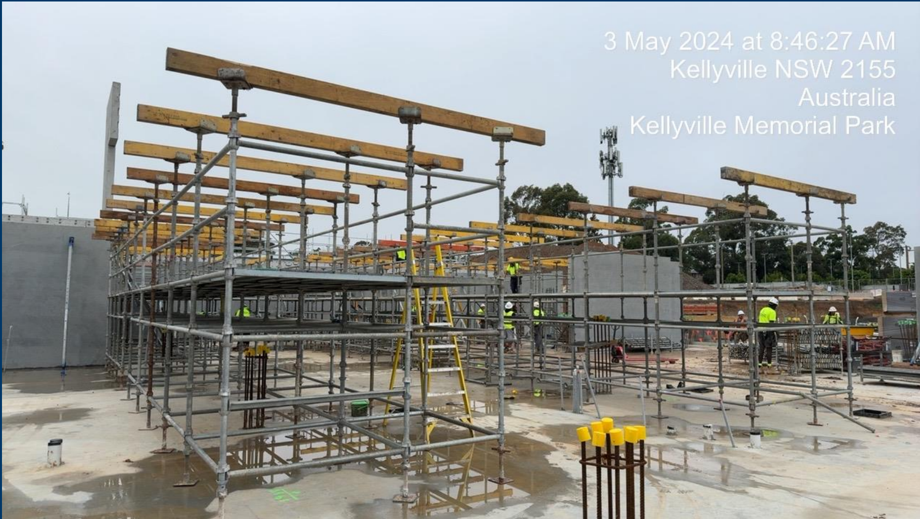
Building B – Upper floor formwork installation
