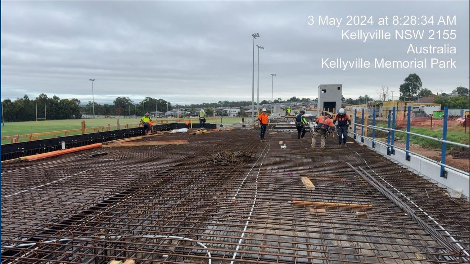
Building A – Steel fixing to suspended deck
